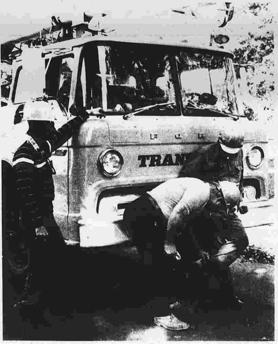
Three electrical workers from Montreal, Quebec, Canada, prepare to go to work this morning at Spruce and Maple streets in an effort to restore power to some of the areas hit by outages on Friday. From left are Willie Marchand, Yves Villeneuve and Jean Guy Methot. The three arrived in Connecticut Saturday morning after Northeast Utilities called for additional help.
