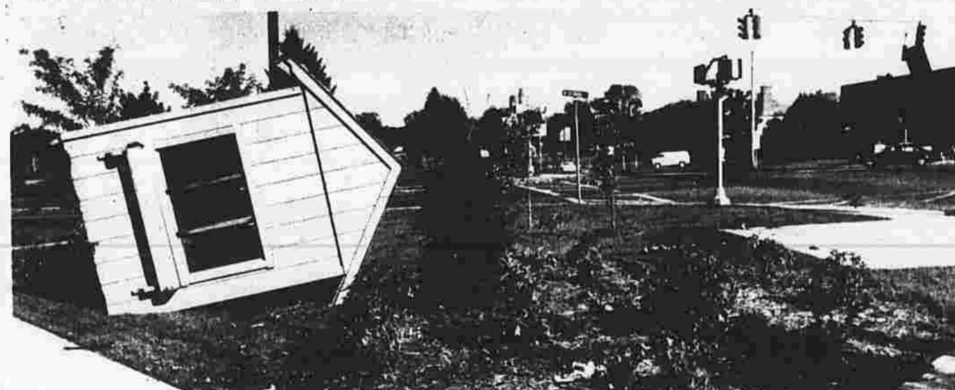
A bus shelter in front of the Mayfair Gardens housing complex at Main and North Main streets lies on its side Sunday after failing to survive Gloria's winds Friday. Despite a large amount of property damage, no injuries were reported in Manchester during the storm.
